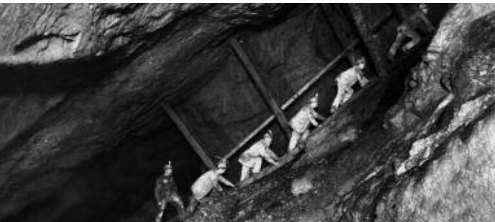
Ladderway at Dolcoath Climbing a flat ladderway is more tiring than climbing a vertical ladder. RIC Archives
