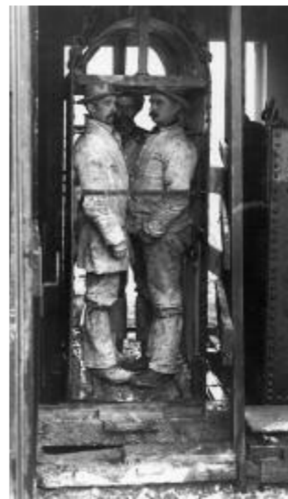
Safety cage - South Conduarrow RIC Archives
